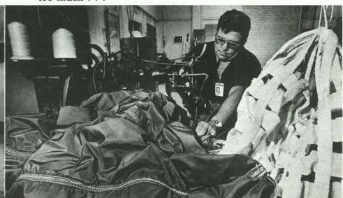
RESEMBLING a huge petticoat, this full scale B77 chute is grappled with by Dennis Cronin as he sews lifting liner onto canopy. Largest chute handled in Lab measured 36 feet in diameter.
